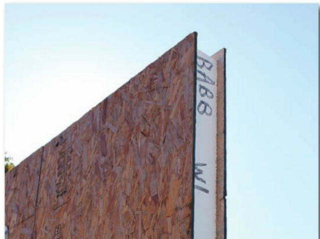
Structural insulated panels are made of wood sheathing laminated to a rigid insulating foam core. Photo credit: Premier SIPS by Insulfoam
