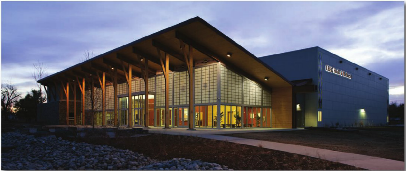
Montana's Little Big Horn College Health & Wellness Center relies on SIPs for energy efficiency Photo credit: J K Lawrence Photography, Courtesy of Springer Group and BNIM Architects
